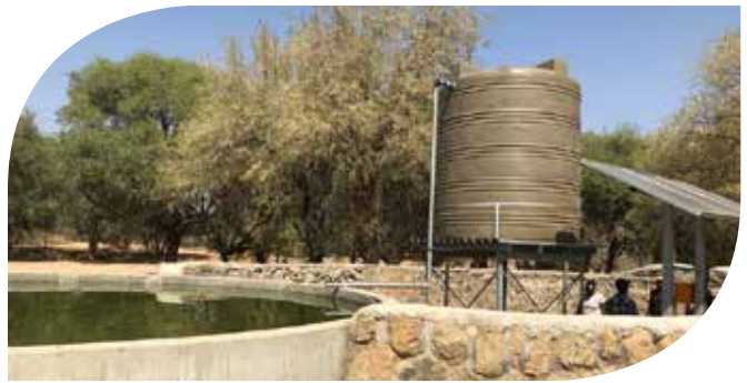
Rehabilitated Borehole under the CBNRM EDA project in the Kunene Region
