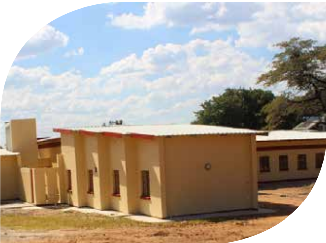
New look for the renovated hostel
