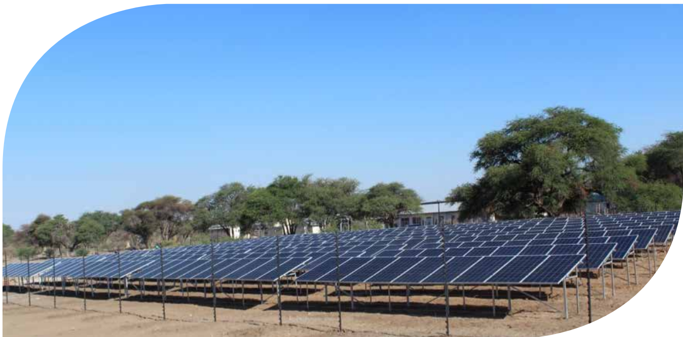
Completed Solar Photo Voltaic (PV) System MCRACE
