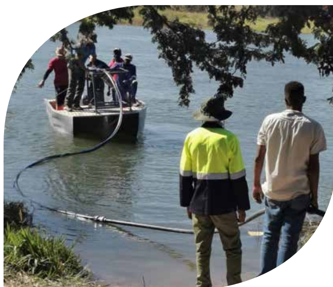
Installation of Solar Water Pumps (SWP)
