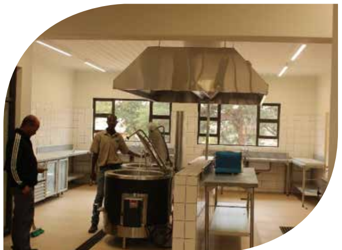
Testing of installed kitchen equipment
