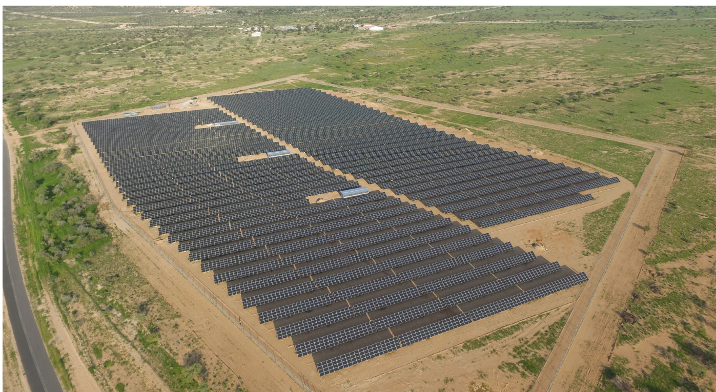
Solar power plant in Karibib financed through the SUNREF Programme
