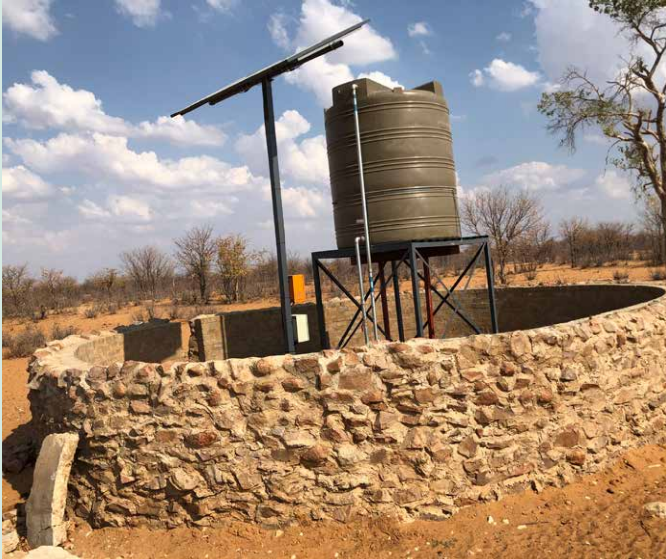
Example of rehabilitated and elephant-protected borehole in the Uukwaludhi Conservancy.
