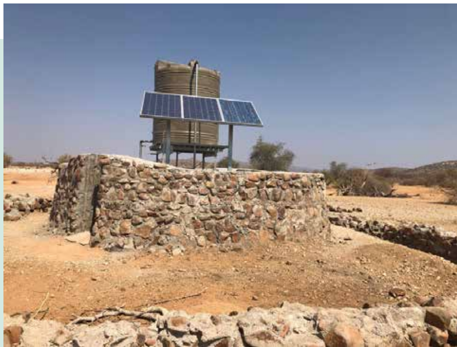
Borehole rehabilitated with solar panels, water tank, elephant protection wall and elephant tank at Makalani Pos Water Point in #Khoadi //Hoas conservancy.
