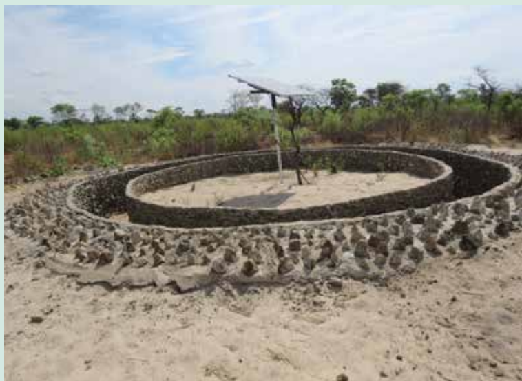
Example of predator-proof kraal constructed at Torra Conservancy in the Kunene Region.
