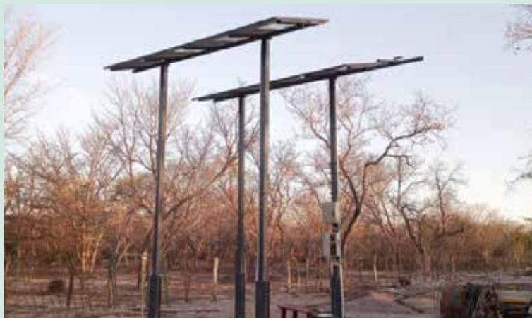
Erection of solar panel stand and installation of the panels for the borehole.
