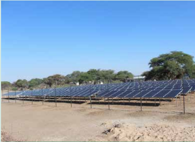
380x130kw PV Solar Panels installed at Mashare Agricultural Development Institute (MADI).
